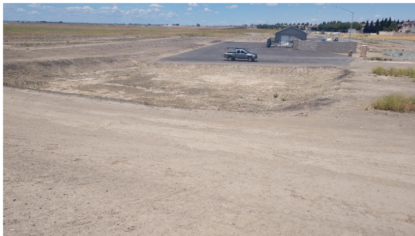
Figure 2 – View of expanded lift station and associated improvements previously within the proposed project Site, looking northwest from the levee .
