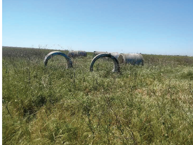
Figure 11 – View of concrete irrigation pipe north of retention pond.
