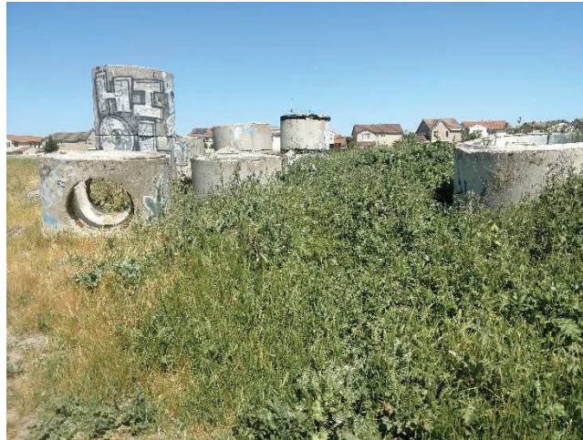
Figure 9 – View concrete irrigation pipe.
