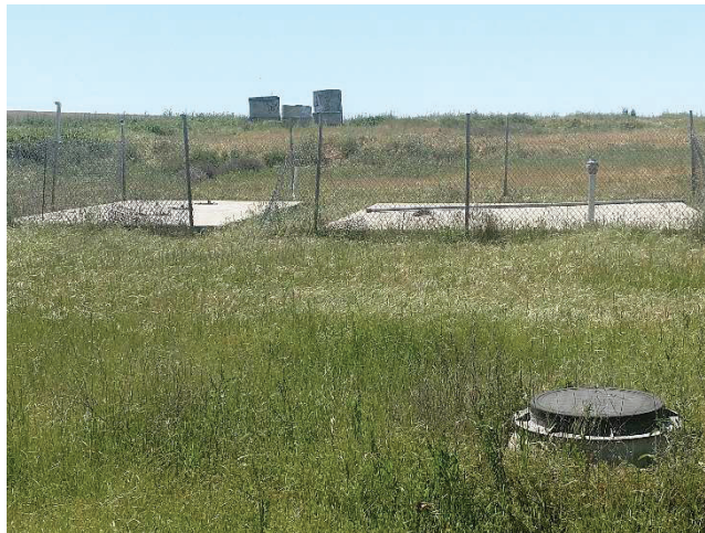
Figure 4– View of concrete slabs and pipe on property adjacent east, looking west.
