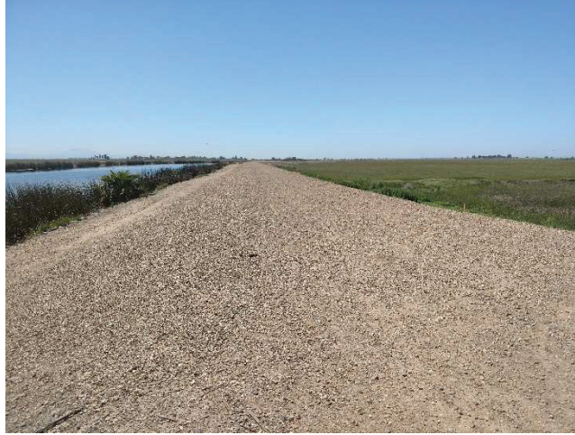
Figure 7 – View of southern boundary, looking west.
